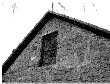
Figure 2. Note the size and arrangement of quarried stones and the area's typical 1890's masonry construction. Original window sills and lintels consisting of single quarried stones. It appears that the roofline has been modified early on, noting fill patterns consistent with the original construction techniques.
