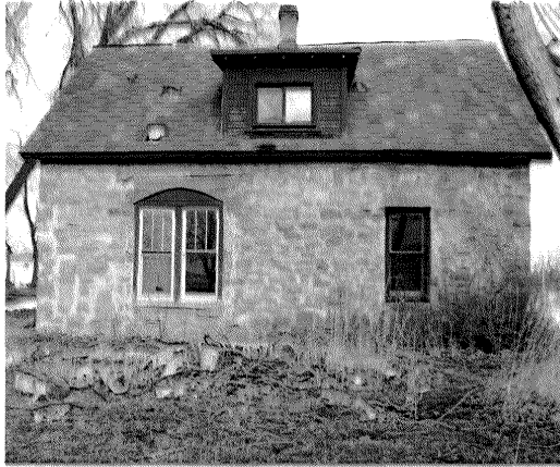
Figure 5. Looking at the south aspect of the house, note the variation of grout coloration, indicative of routine maintenance of the original rock structure. In addition, this photo shows a likely modification to the original house, where the double window likely replaced a single window. The lintel above this remodeled window is concrete and not a single stone lintel as are the remaining windows on the house.
