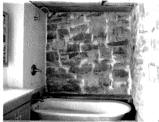
Figure 7. This shows the former exterior wall in the northeast corner, now enclosed inside the added porch. This wall is in excellent condition, having been protected from the elements since being enclosed.
