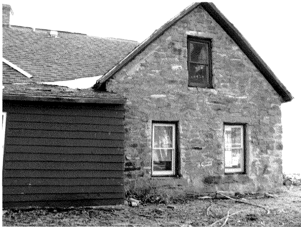
Figure 8. Looking at the western exposed wall of the home. There is an old irrigation ditch roughly 50 feet from this side of the home, and it appears that the proximity to moisture has sunk the southwest corner of the home through the years. There has been extensive grouting of this area, and possibly even newer rocks to replace original rocks that have calved off at some point.
