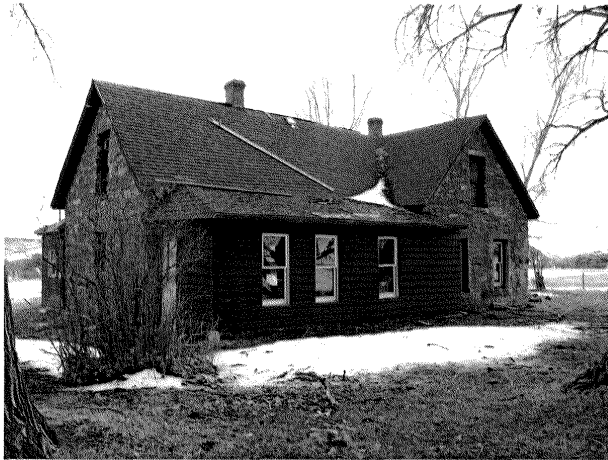
Figure 3. Looking at the north and west sides of the house. The wooden-sided porch is a “newer” addition to the original structure. Note intersecting gable stone walls.
