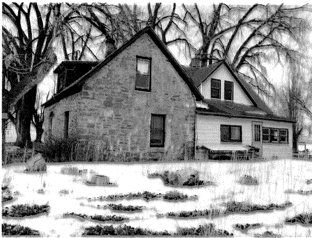
Figure 1. Looking at the south and east sides of present day house. Note the more recent additions made to the original rock structure on the north end. Note intersecting gable stone walls.
