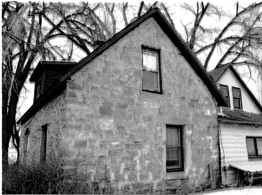
Figure 6. Looking at the eastern aspect of the home. Again, note the roofline that appears to have been extended roughly 6-10" early on in the history of the structure, with different grouting patterns.
